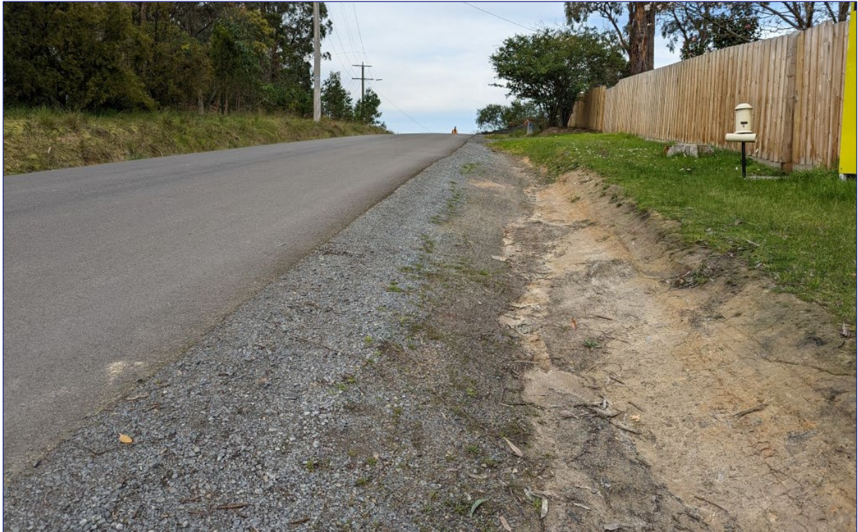
Figure 13: Sight distance towards the south-east - Proposed sight access location (2.5m setback from carriageway)
