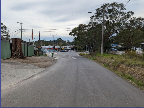
Figure 6: Gear Avenue – view north-west
