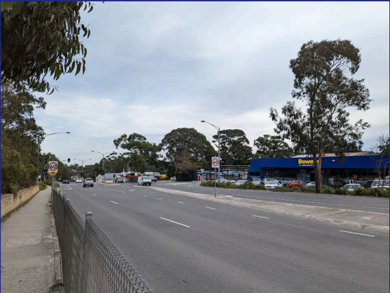
Figure 7: York Road – view south-west
